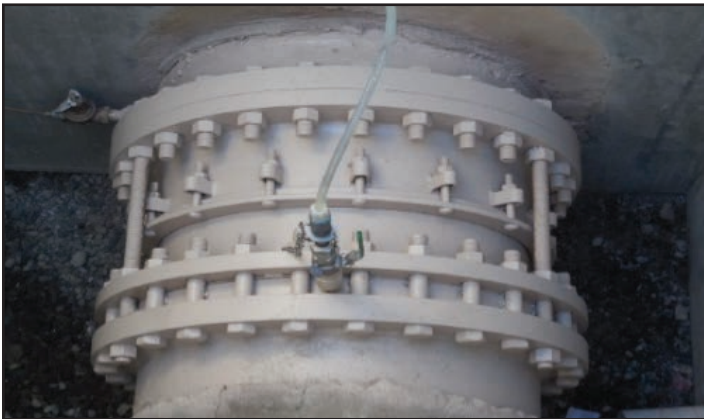
Fig. 5 - 30" wafer mixer installed between flanges
